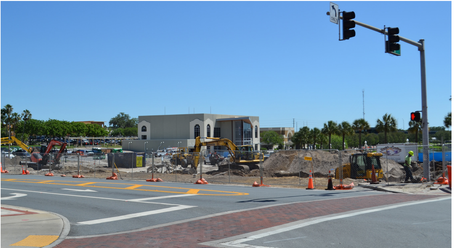
NEW CATAPULT BUILDING CONSTRUCTION (BACKGROUND) AND SUMMIT CONSTRUCTION (FOREGROUND)
